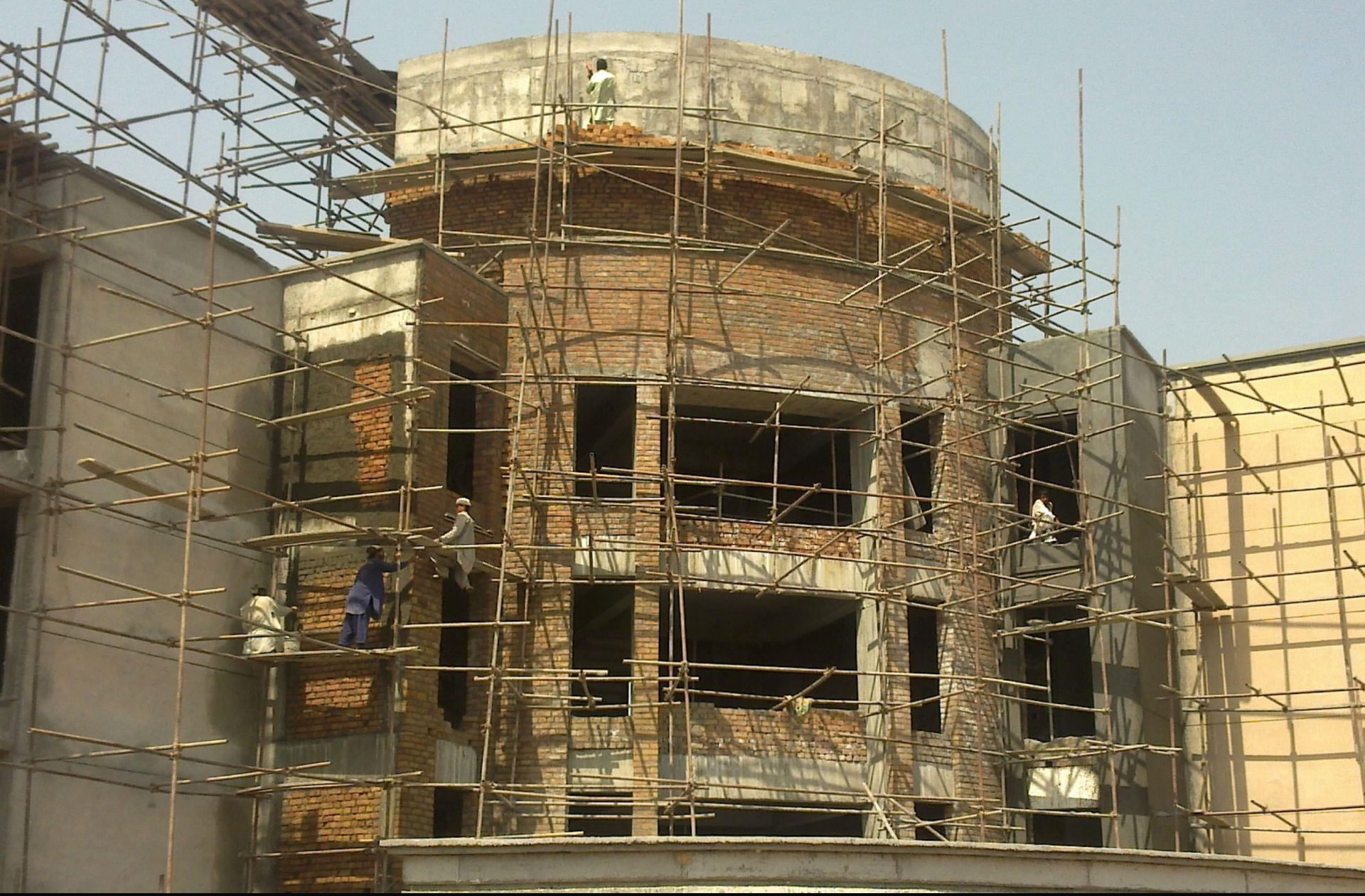
Working at height without wearing Safety Helmet, Safety Harness and Safety Shoes and on unsafe Scaffold platform
