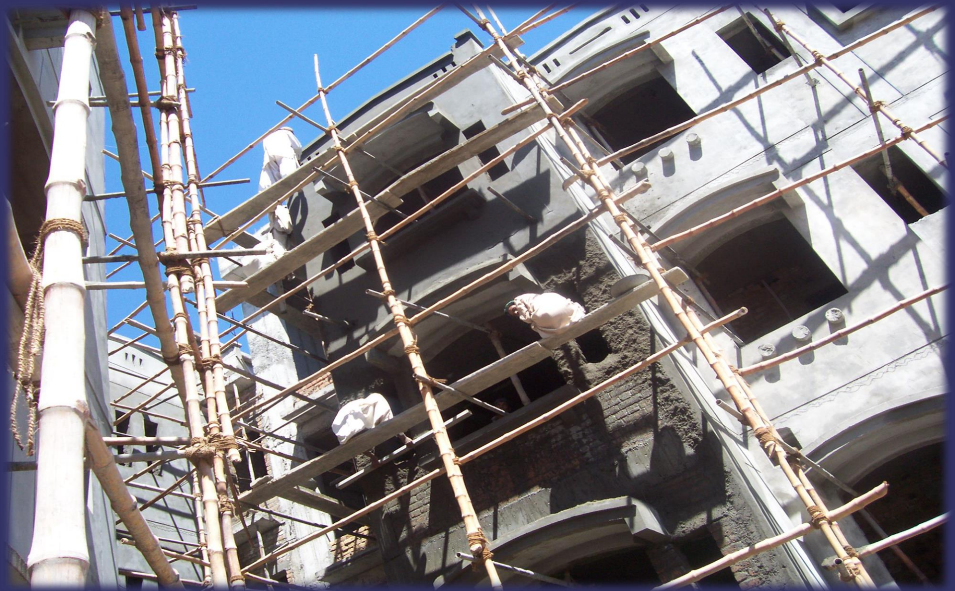
Not proper scaffolding, guard rails, and use of fall protection - personal protective equipment, workers at increased risk
